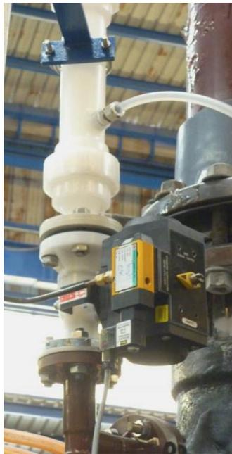
Class 1 PVDF ball valve with pneumatic actuator
